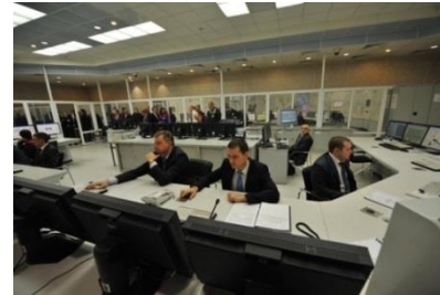
Russia, Rostov NPP Unit 3 - 1000 MW
