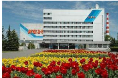
Russia, Kalinin NPP Unit 4 - 1000 MW
