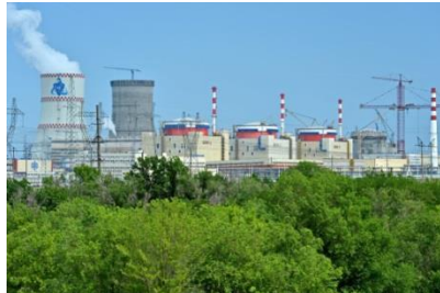
Russia, Rostov NPP Unit 2 - 1000 MW
